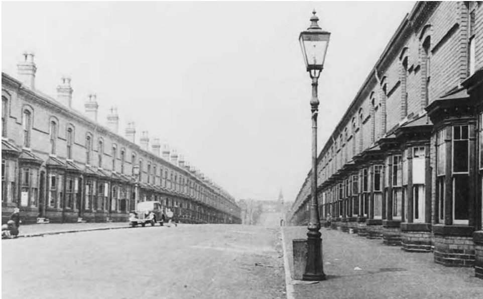
Figure 2.2 Housing built to conform to local by-laws brought marked improvements over the older slums by the last decades of the nineteenth century. The form of most such housing in England and Wales is shown in this 1930s' photograph of Birmingham. Notice the long continuous rows of narrow-fronted houses, built to make maximum use of the wide (and, for developers, expensive) by-law streets, a sharp contrast with the courts and alleys of earlier slums. The houses themselves were larger with better sanitation and small backyards or gardens, giving increased privacy to individual families.
