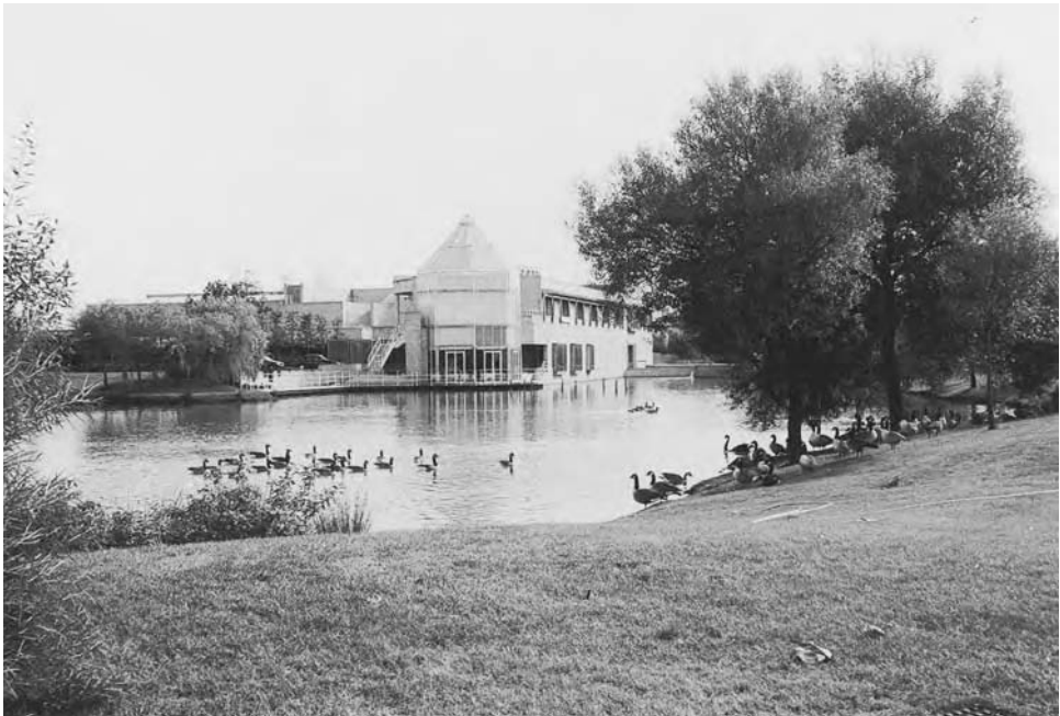
Figure 8.7 Stockley Park, near Heathrow Airport, was one of the new generation of 1980s' business parks, bridging the traditional divide between industry and office activities. It was developed on a former derelict site abutting the inner edge of the metropolitan green belt and offered a superb environment, designed to attract prestige companies.
