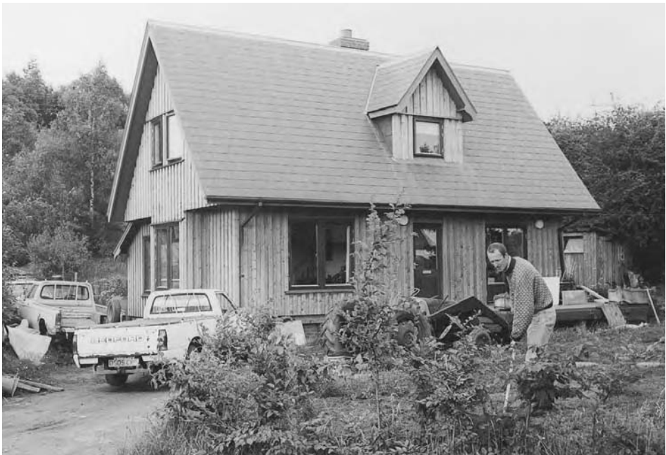
Figure 7.8 Lightmoor, in Telford New Town, was an attempt to recapture the community co-operation of Howard's original garden city vision and harness it to newer concerns for the environment and community architecture.
