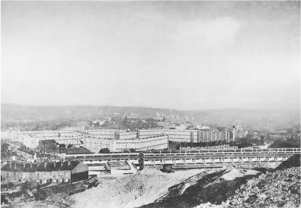
Figure 6.8 ‘Streets in the sky’. One of the main flatted alternatives to the tower block was the deck access medium-rise block. The form was pioneered by the Park Hill estate in Sheffield, visible in the middle foreground, developed from 1957. It was joined within a few years by the neighbouring Hyde Park estate (immediate foreground).
